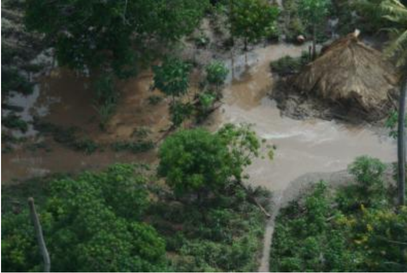
Houses were severely damaged during the floods. Submerged houses in Vila Valdez, Nante. ©INGC 2015
