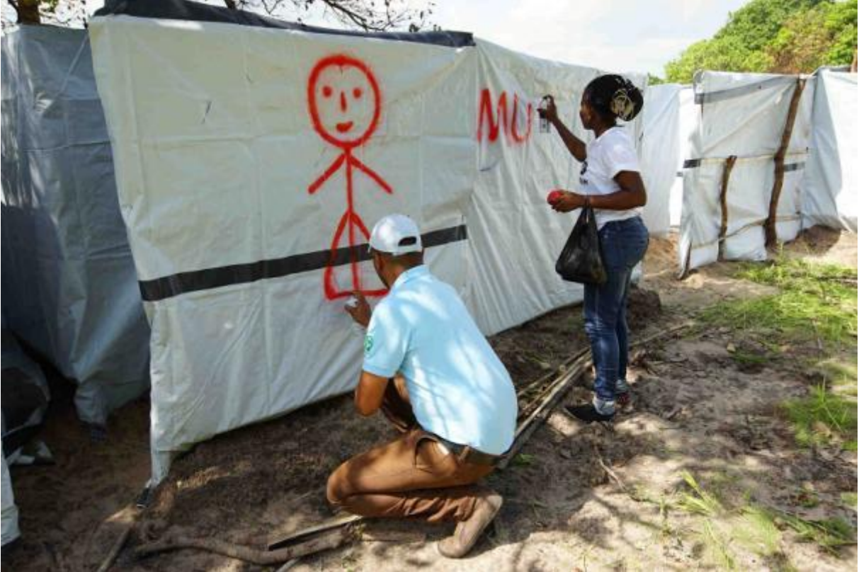
Accommodation centre in Cajual, Mocuba. Latrine construction. ©UNICEF Mozambique 2015 / R. Esmael
