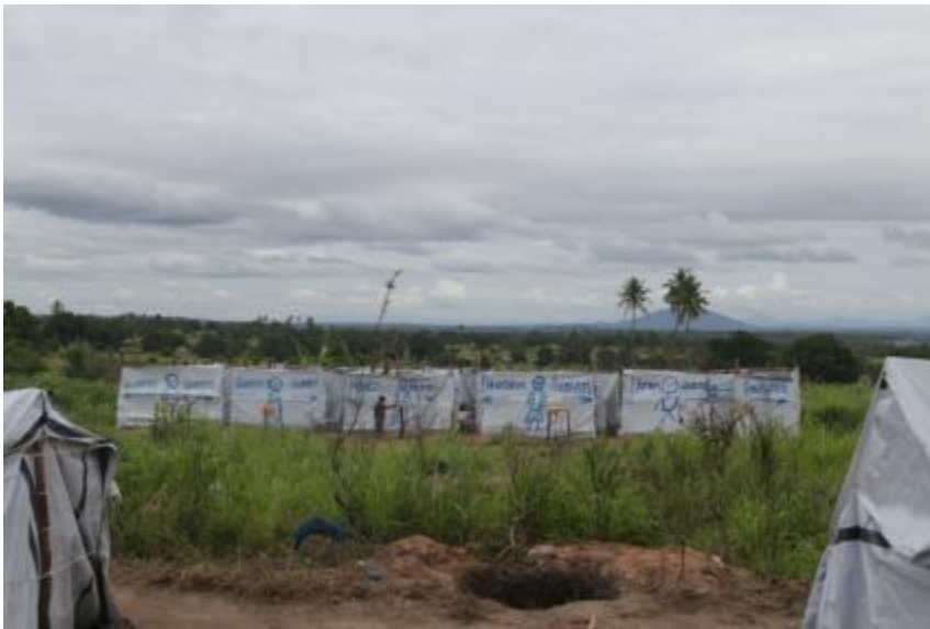
Water, sanitation and hygiene support is being provided to affected and displaced people. Here, latrines built in the Cajual accommodation centre in Mocuba, by partners of HCT and INGC (c) UN-Habitat/Capizzi
