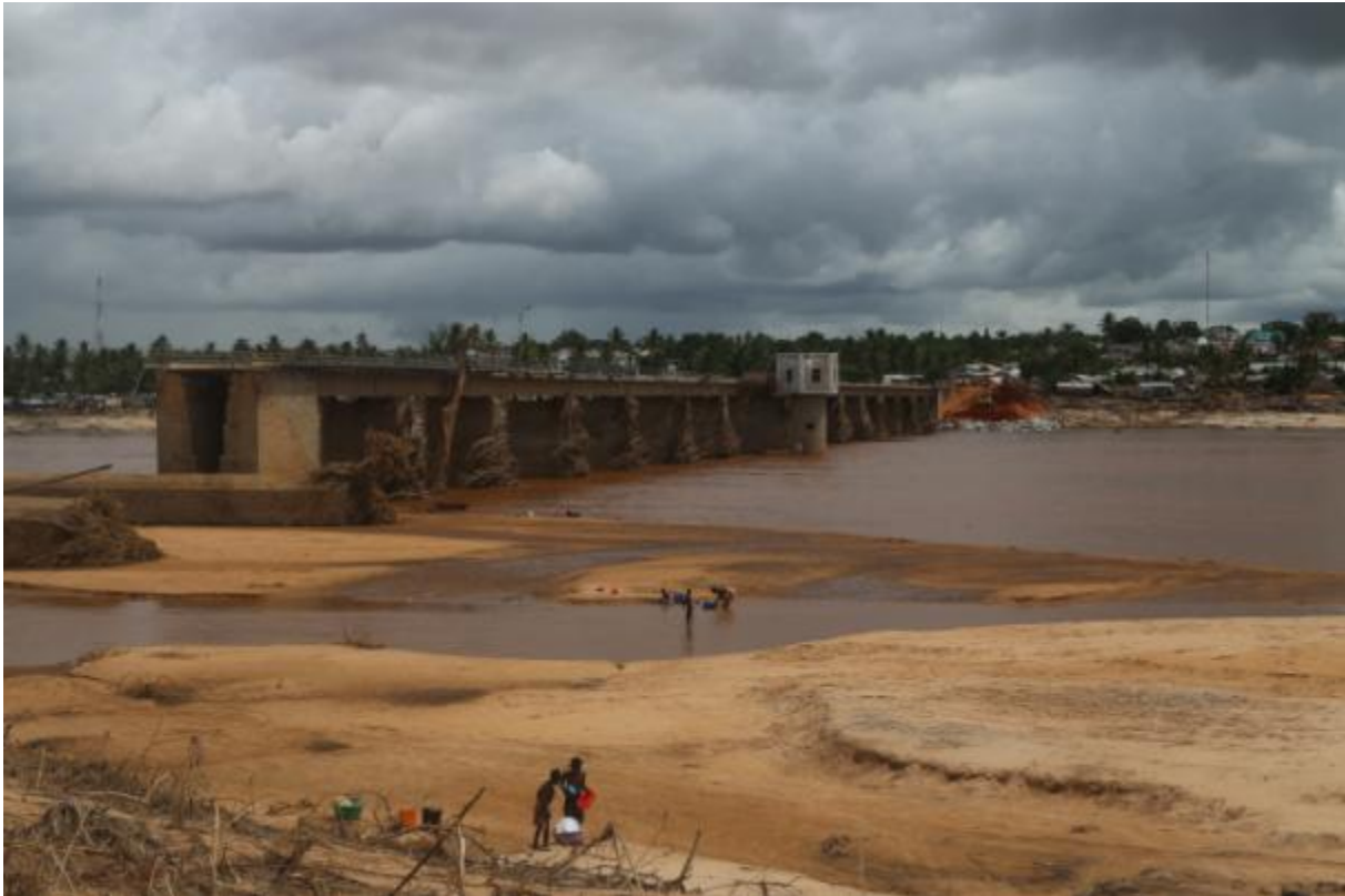
The bridge in Mocuba damaged by the floods cuts the N1 in two, separating North from South of the country (c) UN-Habitat/Capizzi
